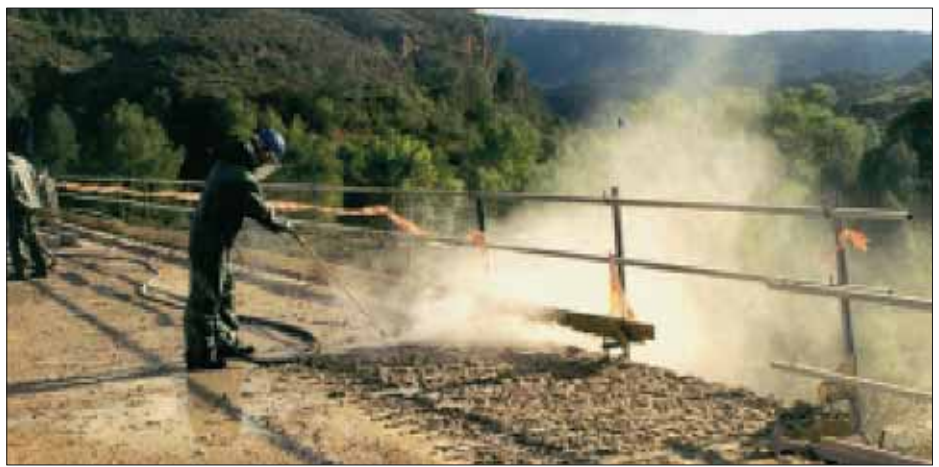
Fig. 5: Hydrodemolition of the existing concrete cover
