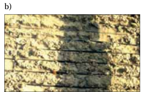
Fig. 3 b): Transverse reinforcement on the existing deck slab
