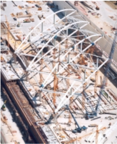
Fig. 5 Erection of the main structure
