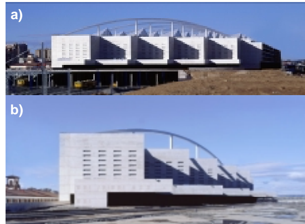
Fig. 2 Zaragoza Delicias station; a) Elevation; b) Façade oblique to the rails, constituted by 5 concrete boxes (Photos by courtesy of C. Ferrater)
