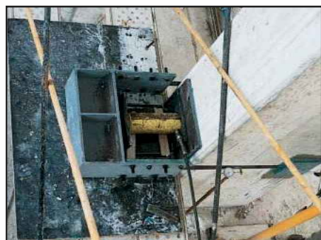
Fig. 6: Field tests for the end anchorage device
