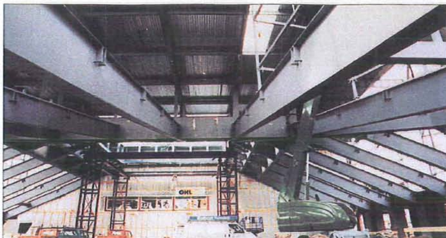
Fig. 6: Upper chord supported on the auxiliary structure during assembly
