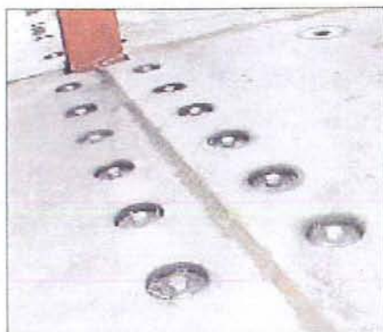
Fig. 3: Composite action of prefabricated concrete slabs and steel girders achieved by prestressed bolts
