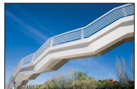
Fig. 8: Stairway constituting the approach span (Photo: Paco Gómez)
