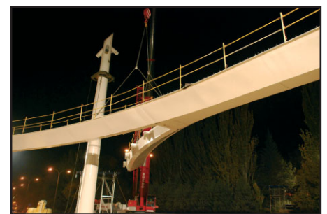
Fig. 7: Erection of main span box girder
