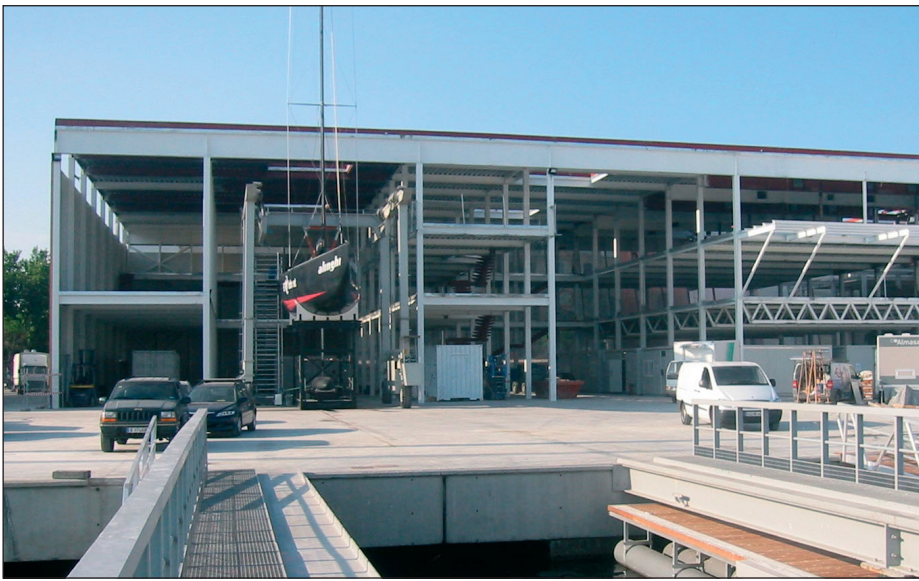
Fig. 2: Alinghi Base during construction, view from the jetty
