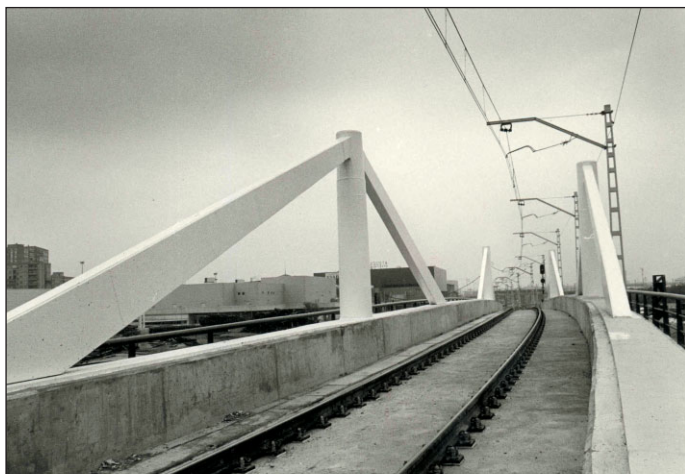
Fig. 3: Top view of the finished bridge
