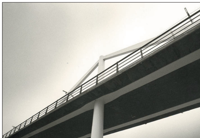
Fig. 4: Under view of bridge deck and intersection with pier
