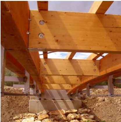
Fig. 10 Esla canal footbridge during construction
