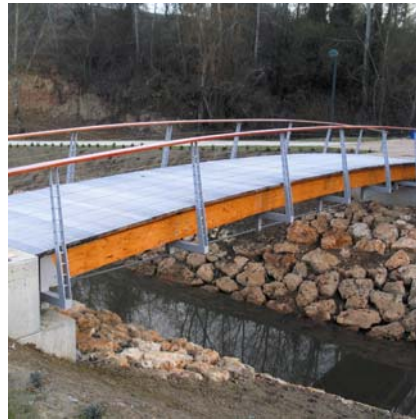
Fig. 11 Esla canal footbridge after completion
