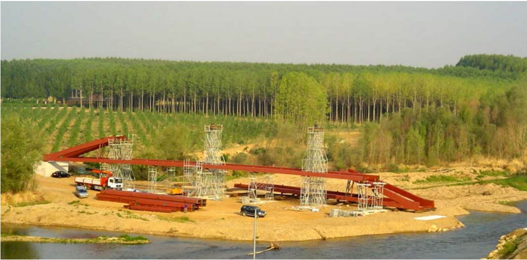
Fig. 5 Provisional artificial island and temporary supports for bridge assembly
