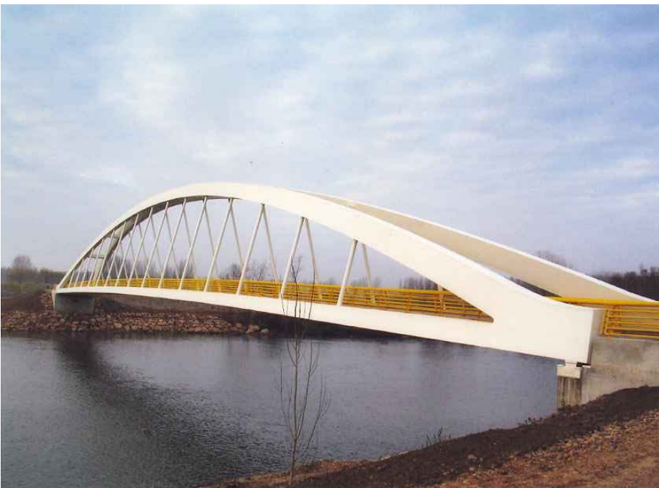
Fig. 6 Esla River footbridge after completion
