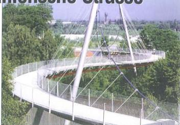
deck at each rib, changing their inclination continuously along the length of the structure, giving users a three-dimensional experience of the structure
